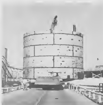
TOWED BY a big "cat" tractor, No. 20 tank moves toward the harbor area to be loaded on a barge. LASTRA DOOR di un "cat" tractor grandi. Tanki No. 20 ta move den direccion di haaf.
